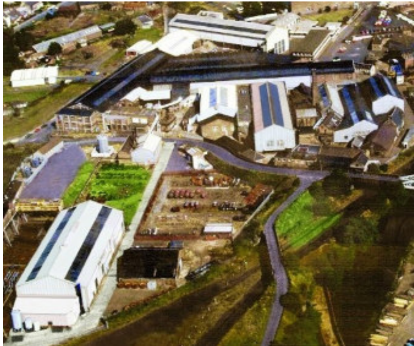
LEVEN, FIFE, SCOTLAND UK FACILITY
