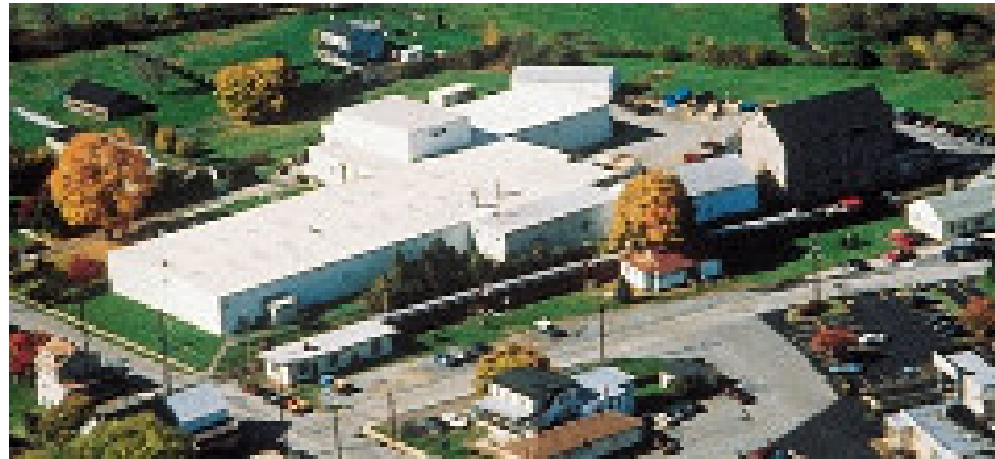
AVONDALE, PENNSYLVANIA USA FACILITY
