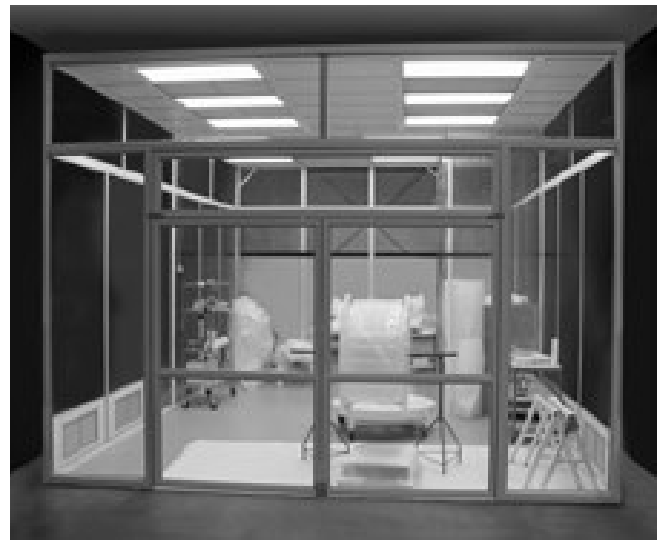
Class 10,000 Clean Room
